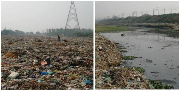
Figure 11: Old Dump Site “How it Looked” Before Work Began
